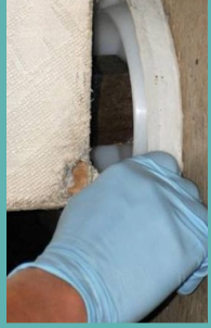
Caulk cracks and spaces
