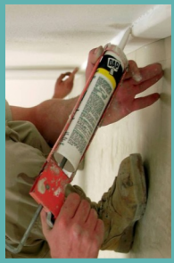
Caulk cracks and spaces
